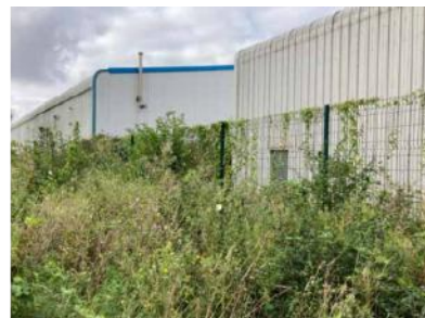
Adjacent warehouses through boundary fence
