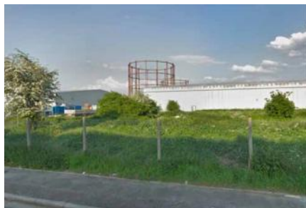
West towards the site from Centurion Way
